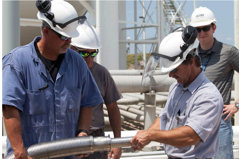
Figure 31. Inspection of an LH 2 supply hose at NASA's Kennedy Space Centre (Photo credit: NASA/Frankie Martin).
