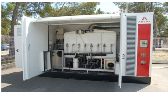
Figure 18. A FC back-up power coupled with IP Energy data centre.
