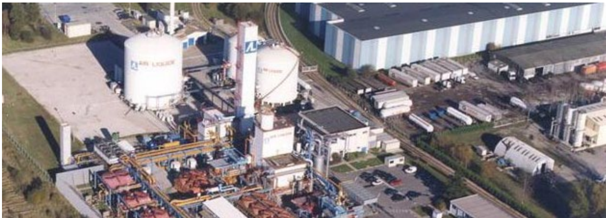
Figura 7. Steam reformer di AirLiquide [1]
