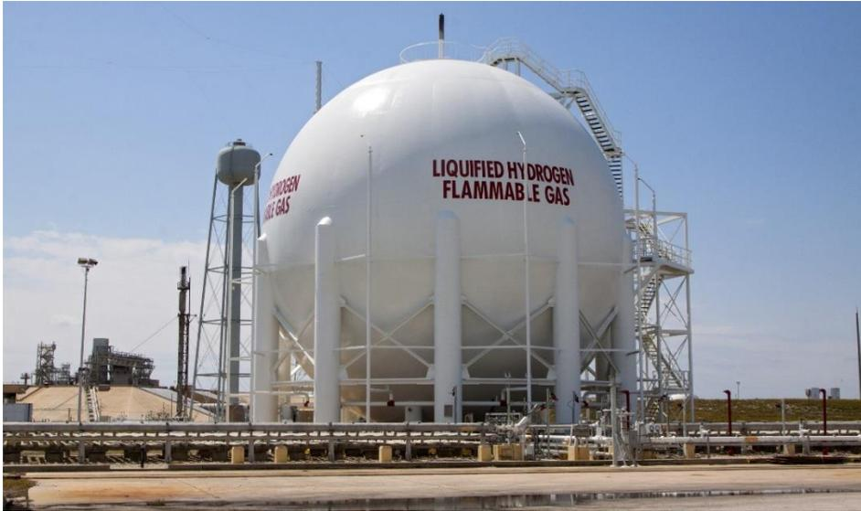
*LH<sub>2</sub> storage vessel with 3800 m<sup>3</sup> capacity at KSC in Florida*
